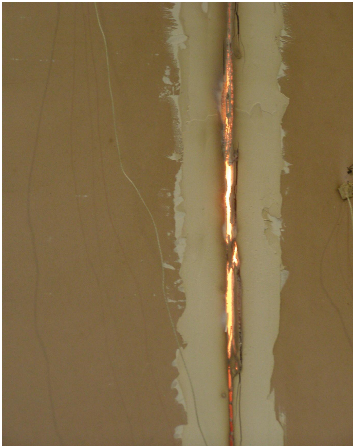
Photo 4 Location of integrity failure (129 minutes).
